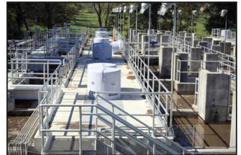
building with improved screening and grit removal machinery protects the plant from harmful materials while a new 1,000 kilowatt generator supports ongoing operations in case of a power supply outage. A computerized Process Control System provides operators with automatic control of all treatment processes as well as monitoring of all
