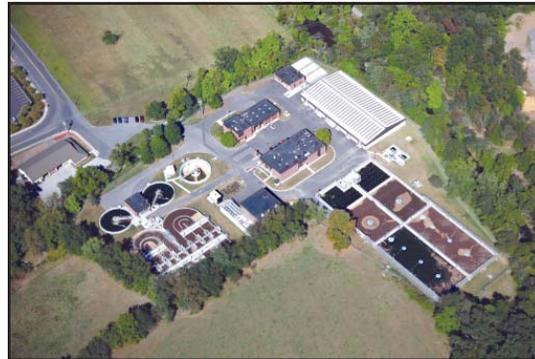
The Gettysburg Municipal Authority's (GMA) Wastewater Treatment Plant was one of more than 160 Pennsylvania facilities required to upgrade in order to comply with state and federal mandated water quality standards. Working closely with their engineer, Buchart Horn Inc., the GMA moved to upgrade processes and expand capacity to 3 million gallons-per-day at its Gettysburg Wastewater
