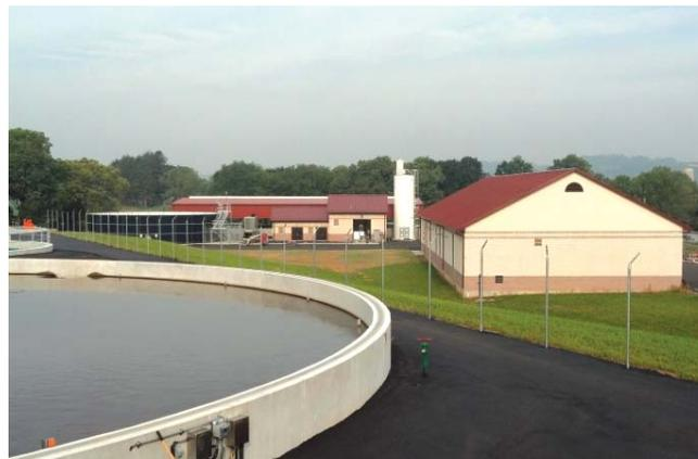
The new facility has a design capability of 1.5 MGD, with a peak hydraulic capacity of 6.0 MGD. As such, process equipment was selected to allow for turndown at current conditions to maximize energy efficiency, while still meeting
